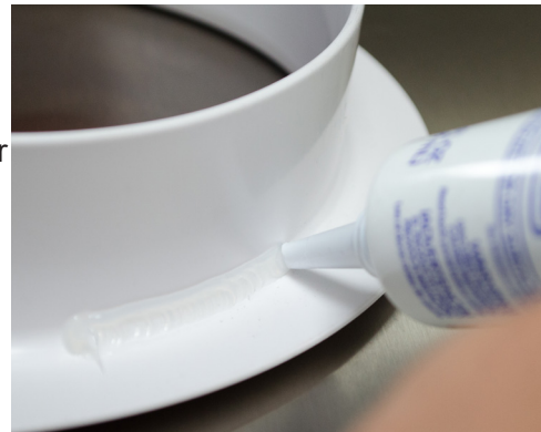
FIGURE 2.24 - Silicone Application
