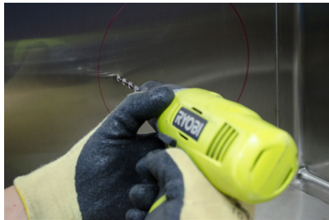
FIGURE 2.10 - Starter Hole
